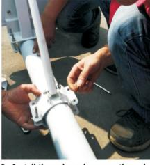
8. Push the butten so switch is on. 9. Install the pole on base, southwards.
